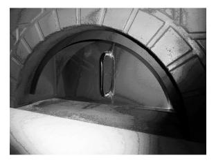
The door is positioned deeper inside when the oven is not working. This way the chimney is insulated from the baking chamber.
